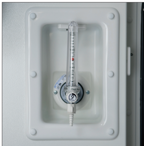
Figure 11.17 Pressure-compensated flowmeter attached to a Schrader outlet.
