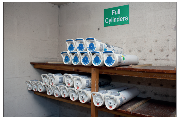
Figure 11.7 An ambulance station medical gas cylinder store.
